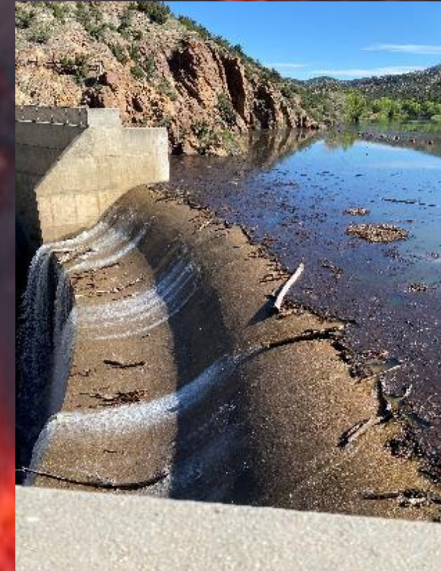
Nambe Reservation, Nambe Dam/Reservoir
